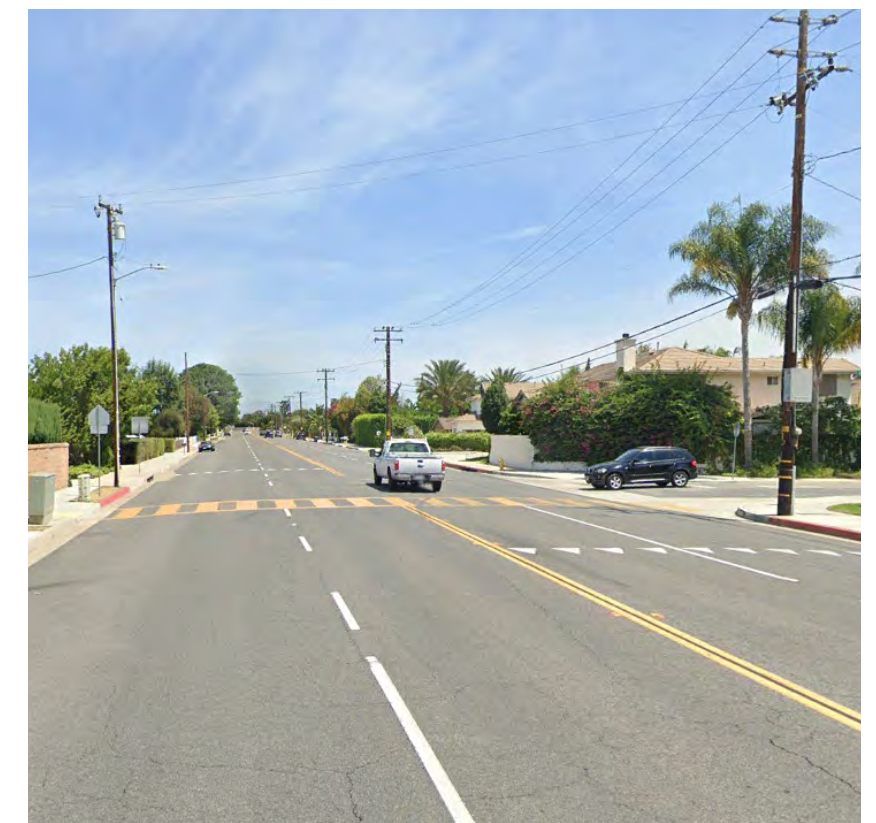
There are two uncontrolled school crosswalks across Holt Avenue
