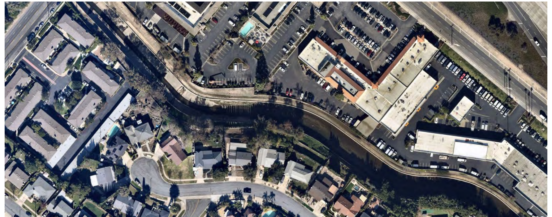
The Santa-Ana Delhi Channel connects to neighborhoods and commercial areas
