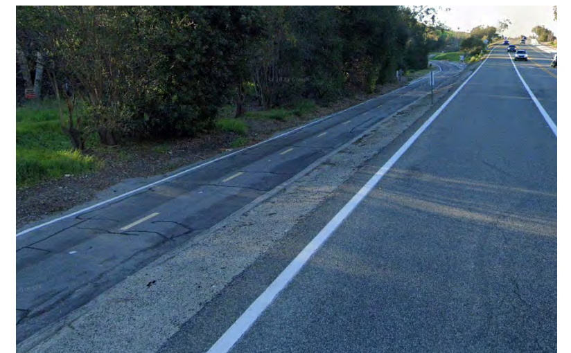
The recommended bike lanes on Live Oak Canyon Road would connect to the existing shared-use path on El Toro Road
