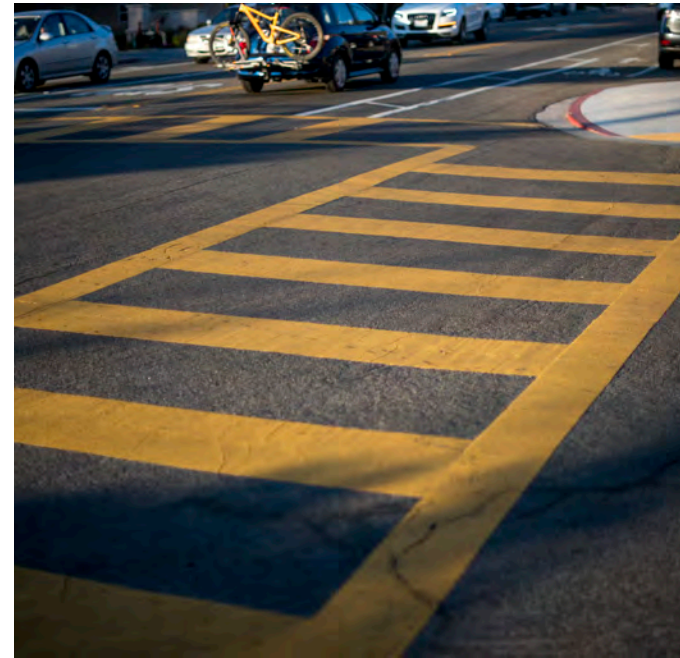
High-Visibility Crosswalks: feature special roadway striping that enhances visibility.
