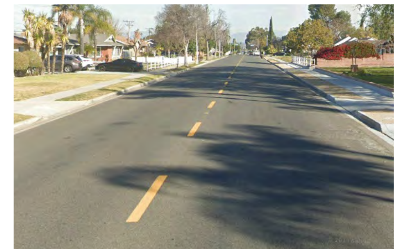
Restriping Segment A can narrow traffic lanes and act as traffic calming
