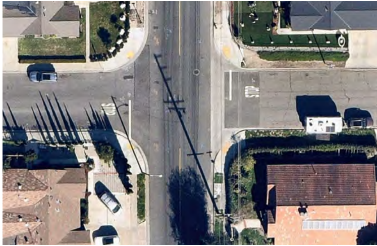
The recommended bicycle boulevard intersects with recommended pedestrian improvements at Hopi Road
