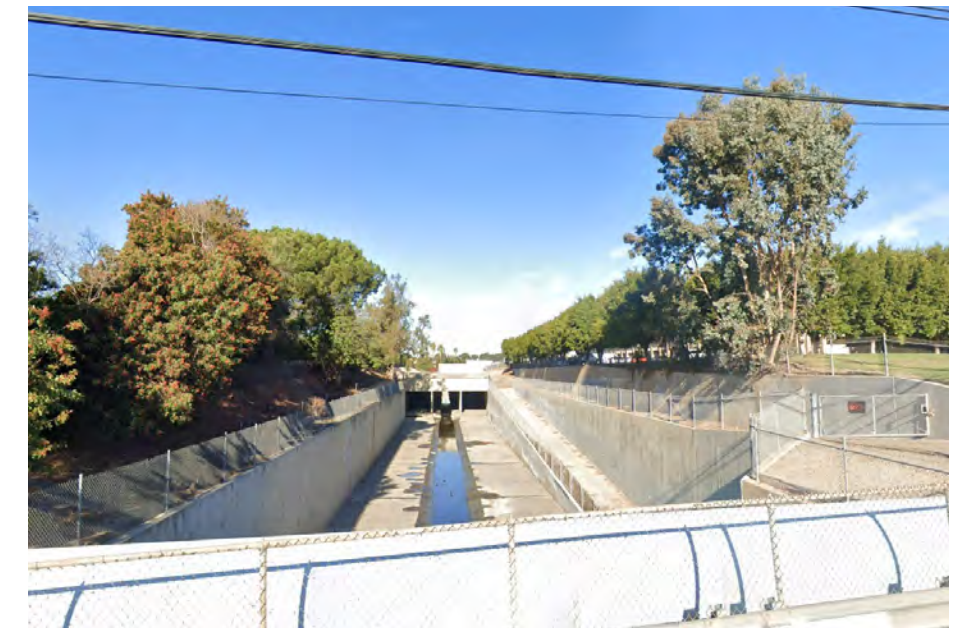
Photo 6: Flood control maintenance road near Costa Mesa in the central quadrant (Figure 102).
