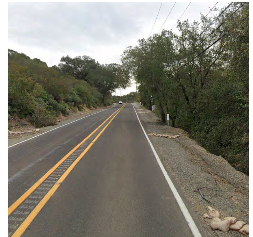
An unpaved shoulder lines Live Oak Canyon Road.
