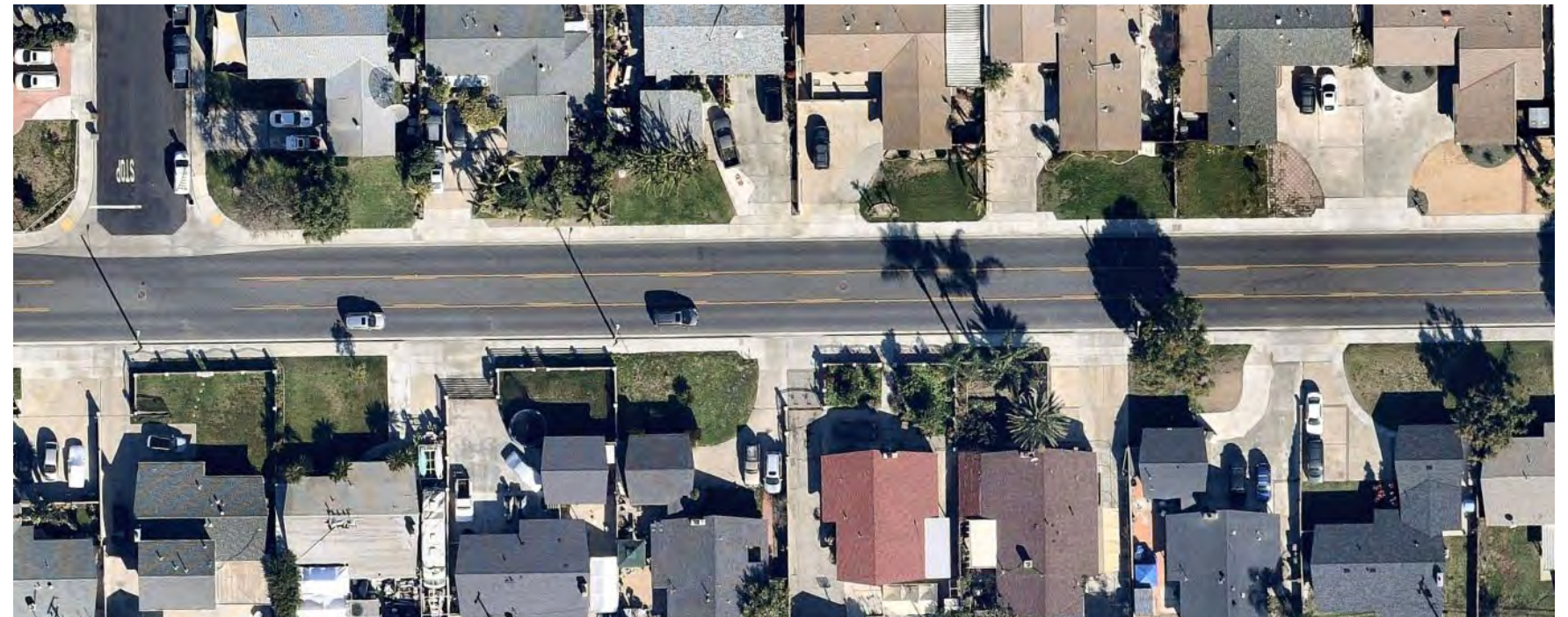
Cerritos Avenue has three traffic lanes, including a center turn lane
