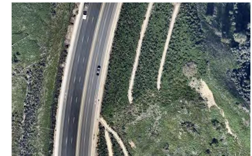
When Antonio Parkway turns into Avenida La Pata, the recommendation changes to a Class I shared-use path
