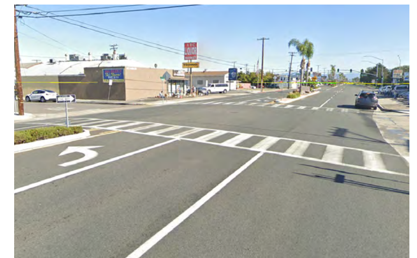
Segment B of Bolsa Avenue intersects with Tier 1 pedestrian recommendations at Jackson Street
