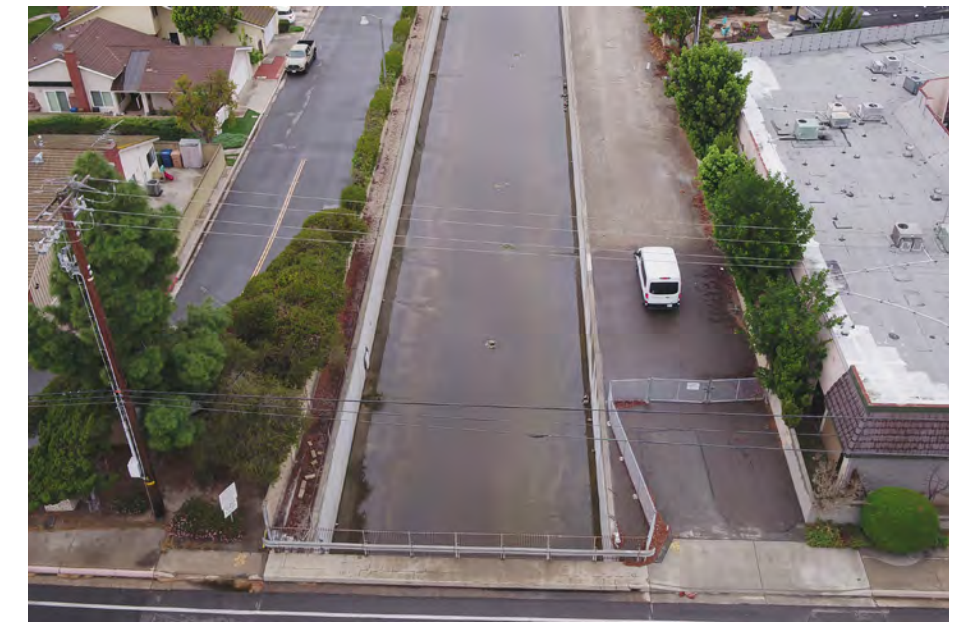
Photo 4: Flood control maintenance road along the Bolsa Chica channel near Rossmoor Island in the northwest quadrant (Figure 101).
