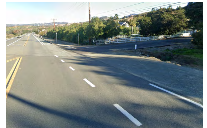
Installing a shared-use path will help reduce conflict points, like here where motor vehicles must cross the bike lane to turn right
