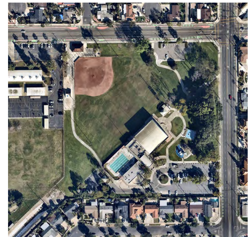
The channel moves underground under Rosita Park and the Salgado Community Center
