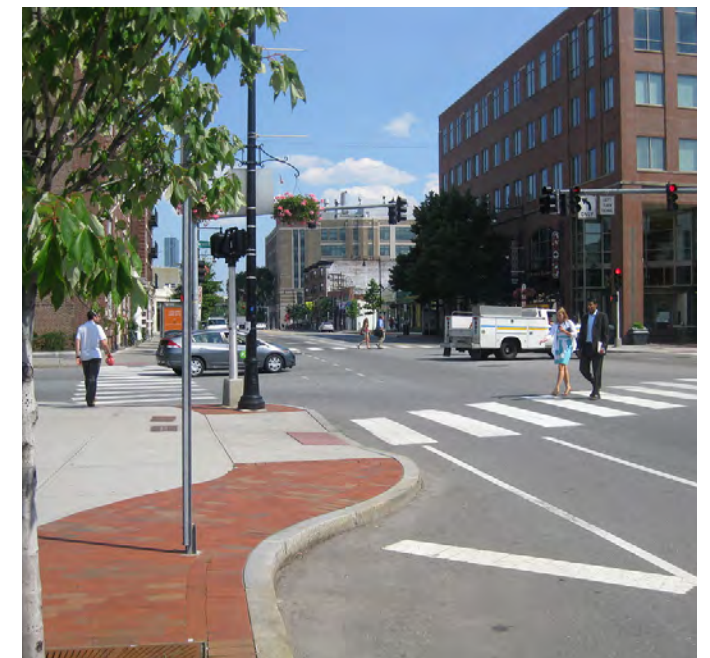
Curb Extensions: are extensions of the sidewalk area that can reduce crossing distances.
