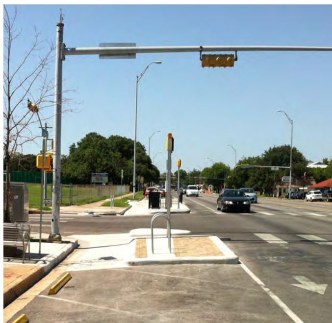
Slip lane Modifications/Corner Radius Reductions: slows turning vehicles and shortens pedestrian crossing distances.
