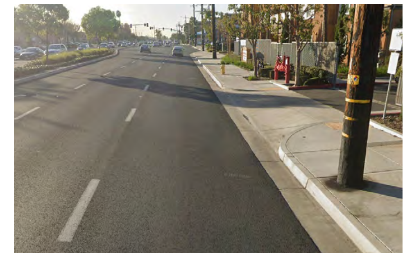
In all segments, a westbound vehicle lane can be removed on Katella Avenue to fit a Class II bike lane
