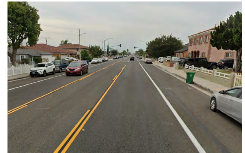
Future design studies can determine if removing the center turn lane, or removing on-street parking is most appropriate for this recommendation
