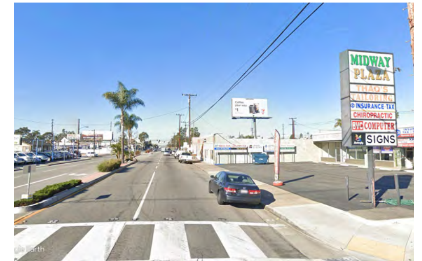
Westbound parking in Segment B will need to be removed to fit a buffered bike lane
