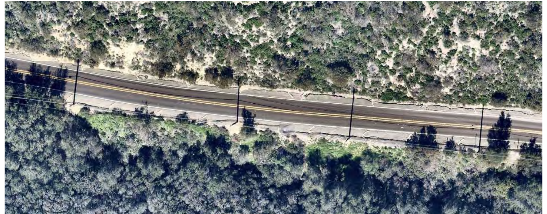
Live Oak Canyon Road is a narrow road with two travel lanes
