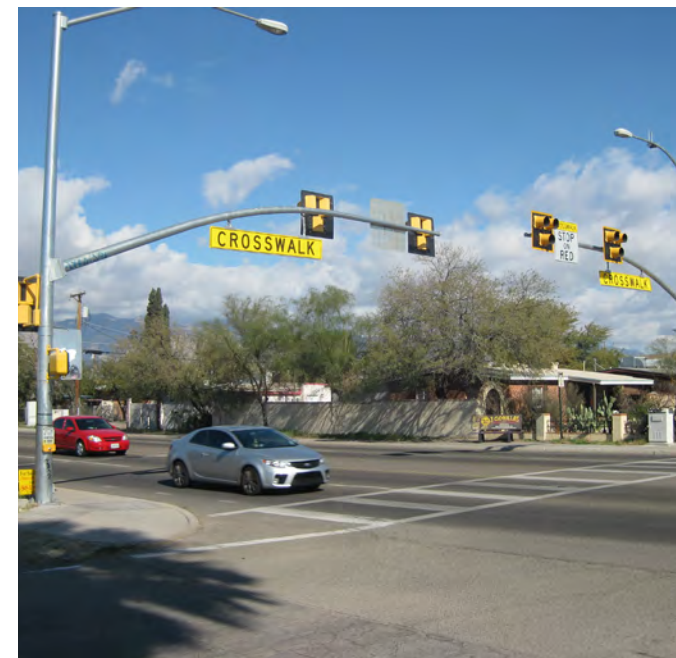
Pedestrian Hybrid Beacon (e.g. HAWK): when activated by a pedestrian, lights overhead turn red indicating that drivers must stop for the pedestrian to cross.
