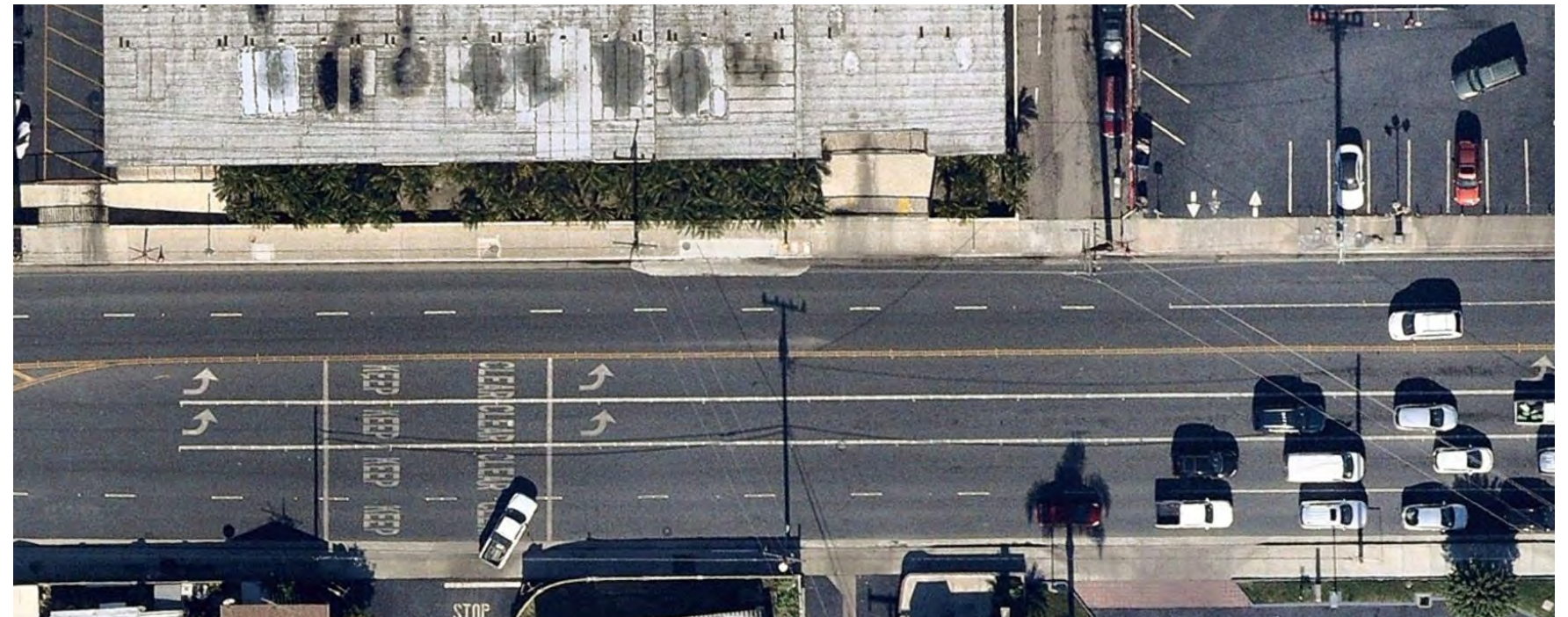
Approaching the Beach Boulevard intersection, McFadden Avenue has six traffic lanes
