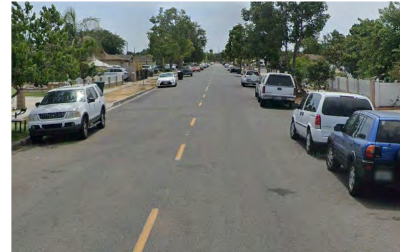
There is a .4 mile portion of Nearing Drive with no controlled stops, which may encourage speeding
