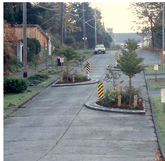
Traffic Calming/ Chicanes: features that reduce vehicle speeds. This image shows chicanes which narrow the roadway to slow vehicle speeds.
