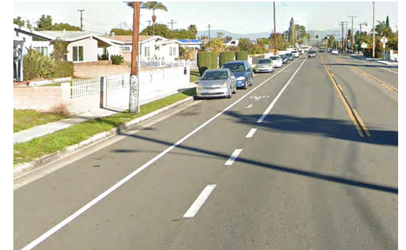
If feasible, the parking lane can be flipped to the outside of the bike lane on southbound Segment B
