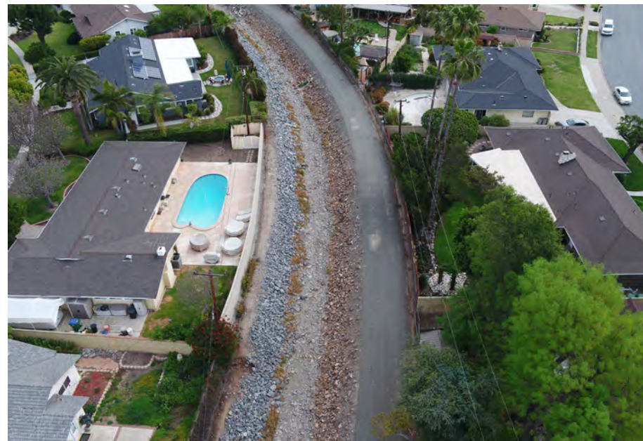
Photo 5: Flood control maintenance road along the El Modena Channel in North Tustin in the central quadrant (Figure 102).
