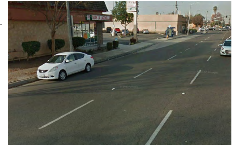
Segment B eastbound parking or a vehicle lane can be removed on Katella Avenue to fit a Class II bike lane
