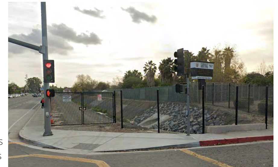
Entry point to Segment A adjacent to Godinez Fundamental High School on St Andrew Place
