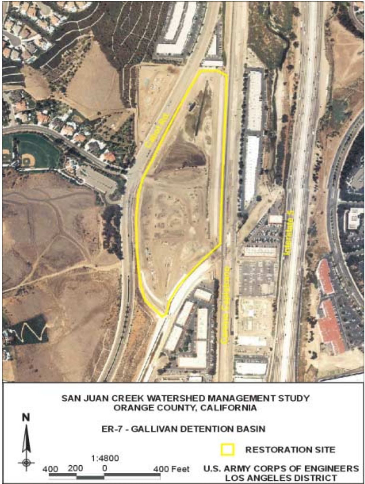
Figure 32. ER-7 Gallivan Detention Basin
