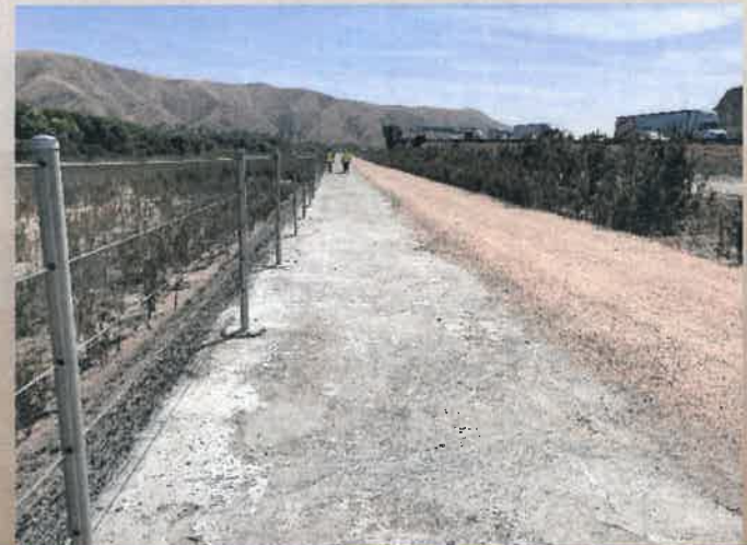
Soil Cement & DG Trail (May 2022)
