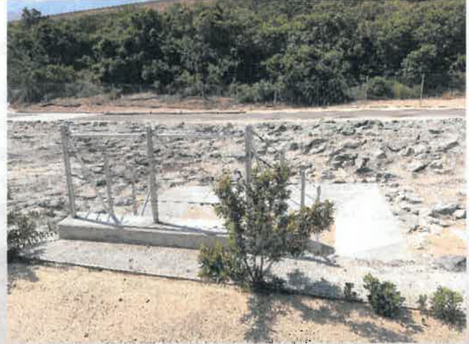
Inlet Structure Adjacent to Bikeway (May 2022)
