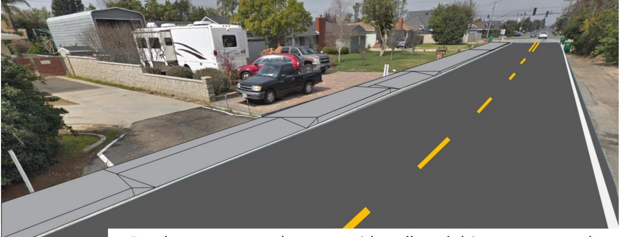
Road pavement, curb, gutter, sidewalk and driveway approaches
